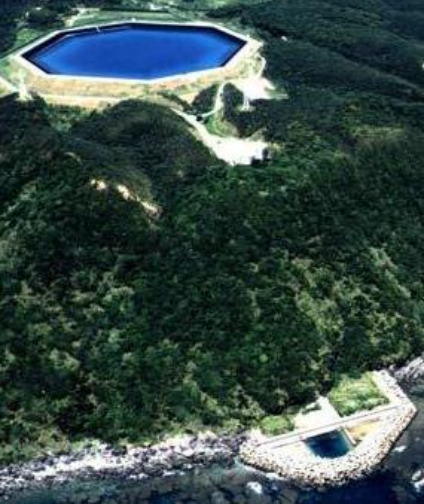
Seawater hydro-electric storage on Okinawa, Japan
